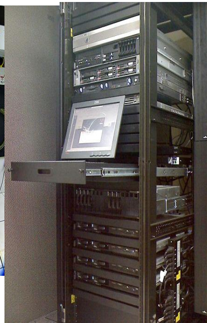
Rack used in Data Centre to house equipment (server, switch, storage )
